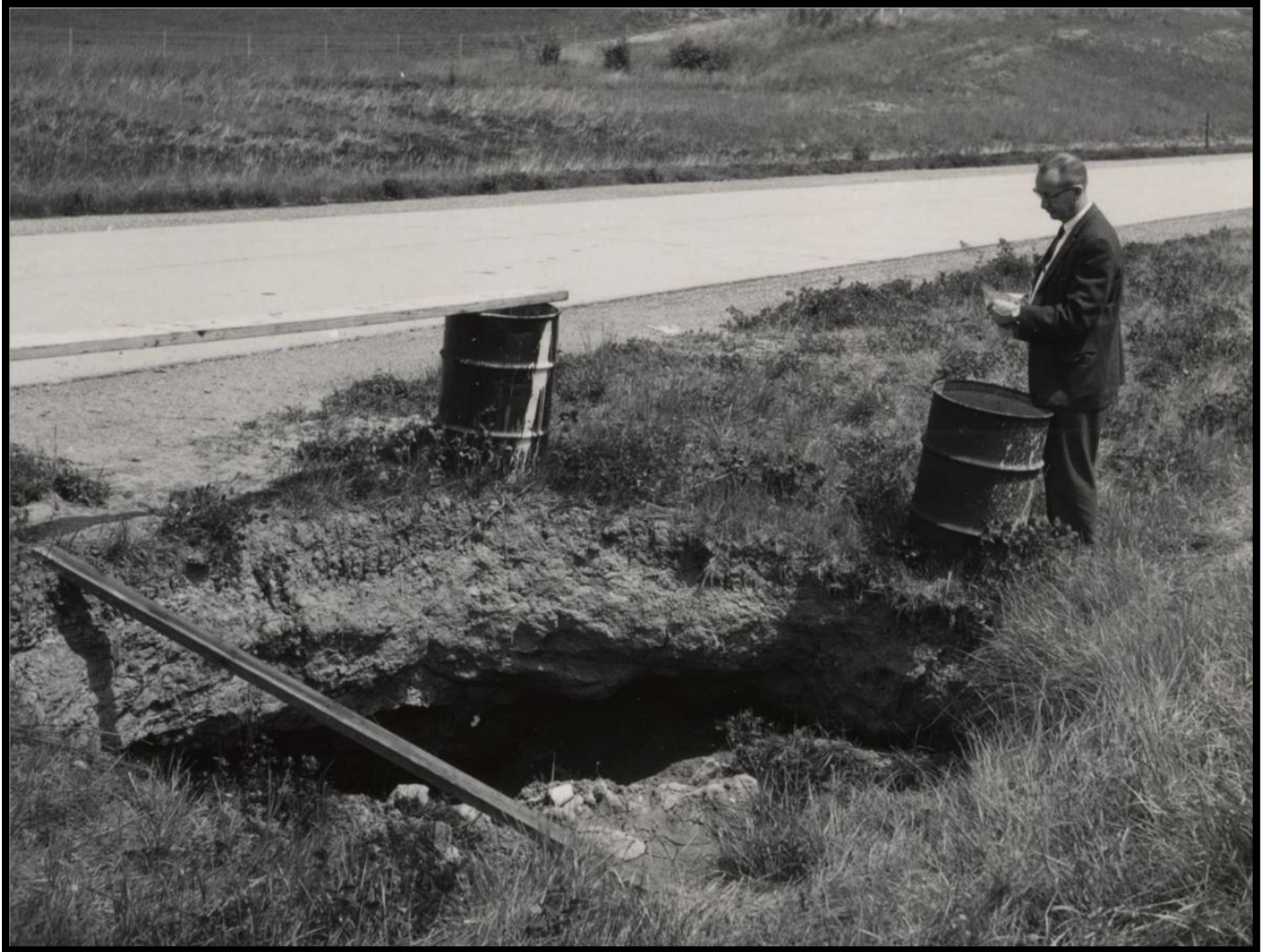
Figure 9. Image of sinkhole resulting from underground coal mining in Ohio. Image from Norell (1970).
