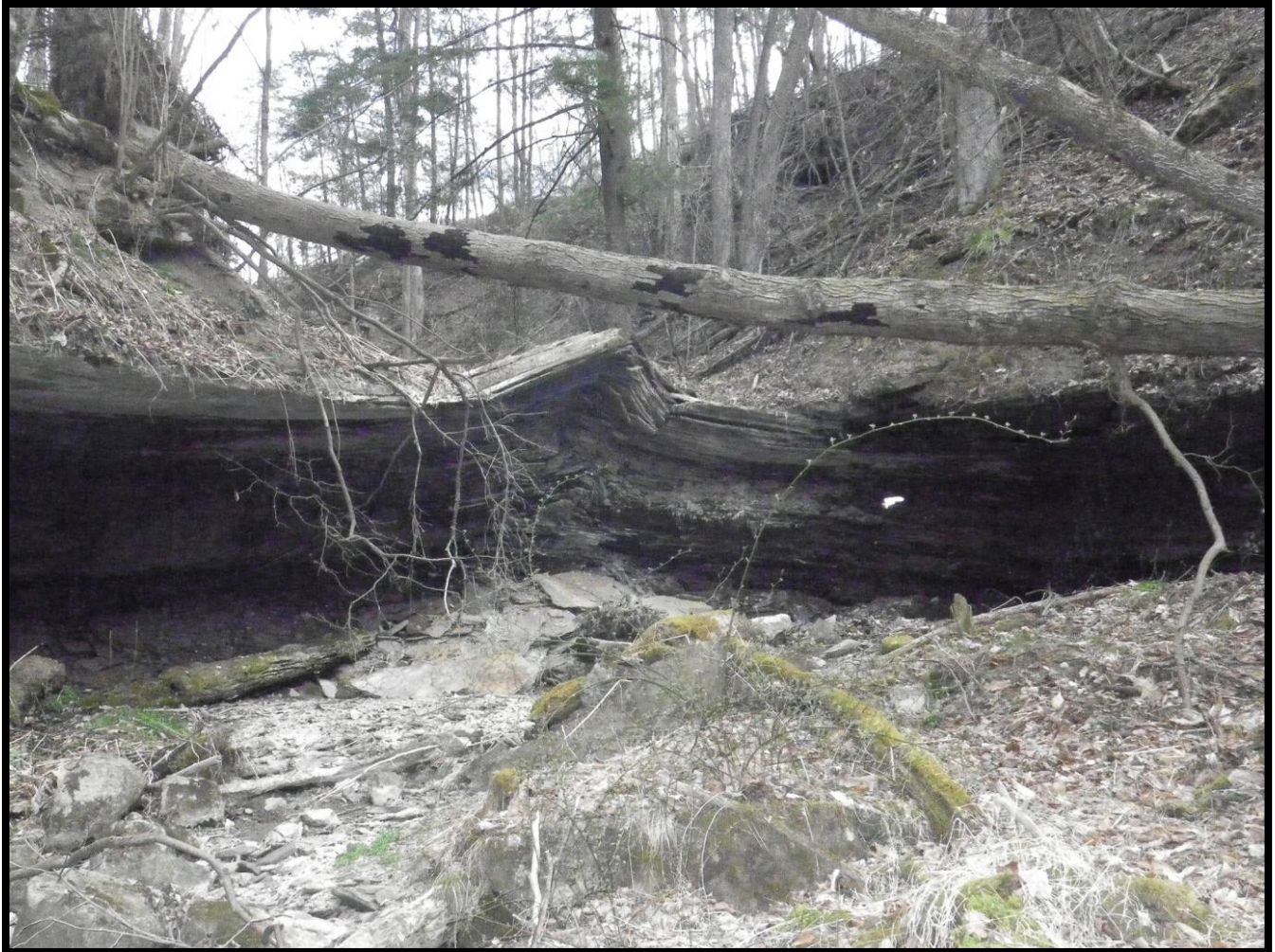
Figure 17. Heave feature, from mining subsidence, in bottom of unnamed tributary of Wheeling Creek located in northern study area. No scale is available for this image; however, the tree that has fallen over likely measures about 1-2 feet in diameter. Image courtesy of Steve Ball, WVDEP.
