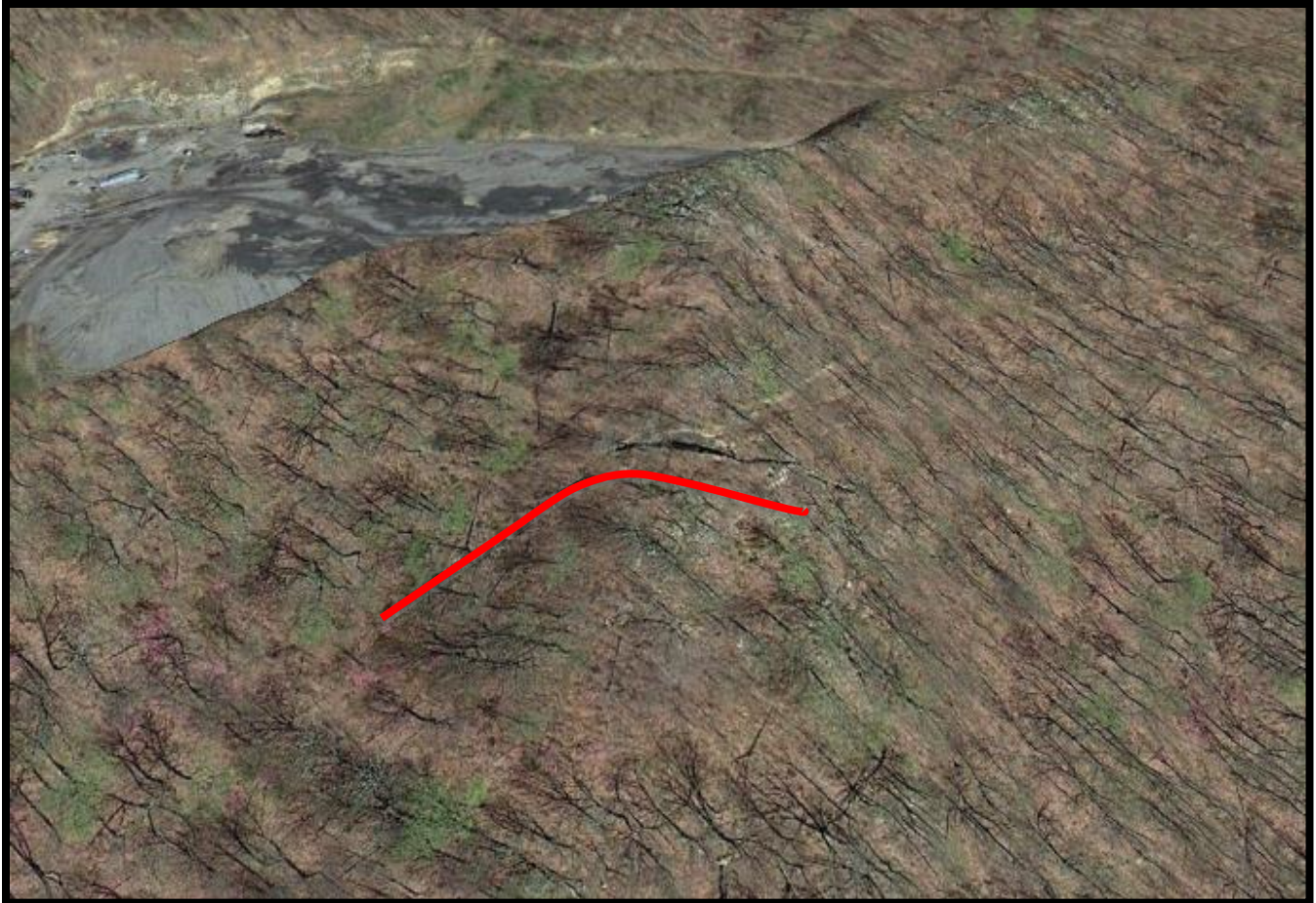
Figure 19. Oblique aerial view of ground crack that measures about 300 feet (91 meters) long (above red line). Crack is located in the southern West Virginia. Coal mining surface operation can be seen in the background. The parallel/repeating sets of black lines in the image represent tree shadows. Image from Google Earth.
