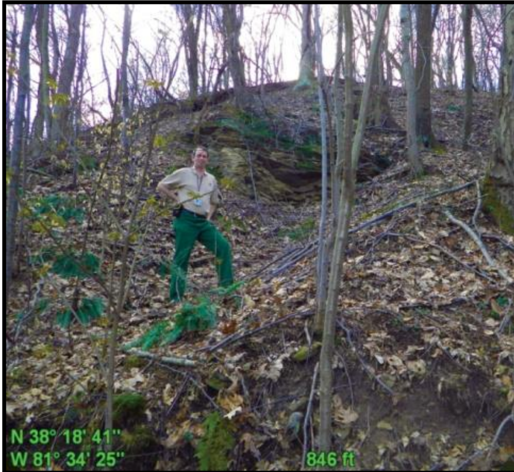
Figure 13. Photograph of portal collapse (location A in Figure 11). Nick Schaer, WVDEP standing immediately downslope of a portal collapse. The portal collapse is indicated by the approximately 5-foot step and zone of convergent topography below it.
