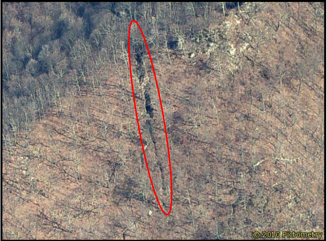
Figure 20. Oblique aerial image of a linear fissure in southern West Virginia. About 300 feet (91 meters) of the fissure is visible in this image. The fissure measures about 15 feet (4.5 meters) at its widest. Three underground coal mines are located beneath this fissure. Image from Pictometry.
