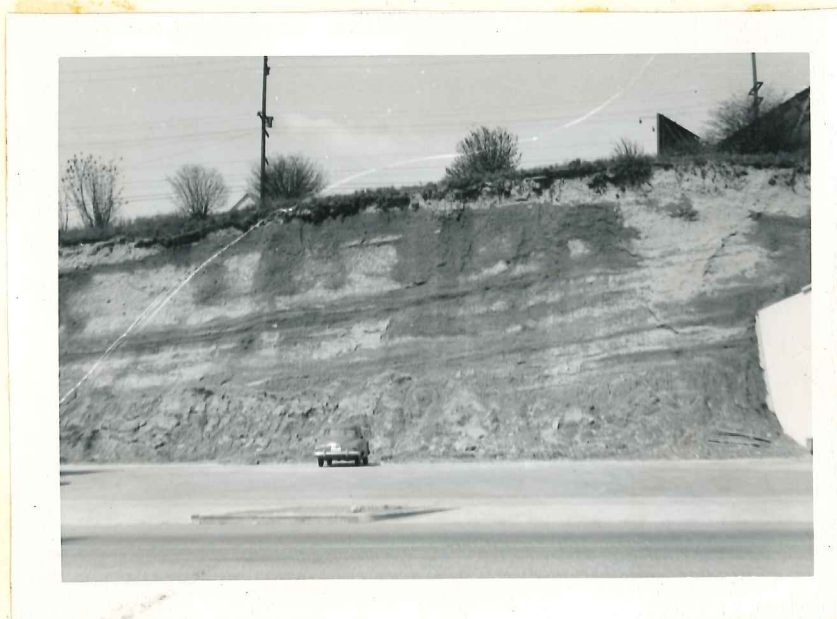
Figure 9. SHEETING IN GLACIAL TILL. Apparent bedding in photograph is structure due to ice movement.
