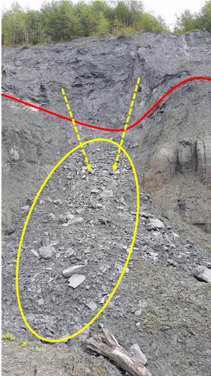
Figure 12 – Photo of a clay/silt block failure along the eastern wall within Lobe 2 of the GBLC. During my field investigations I observed a large block of silts and clays fall from the wall above the red line, then land and crumble as it was deposited within the gully outlined by the yellow circle. The face of the cliff is ~50m tall. The photo is facing east along the eastern extent of Lobe 2 (Figure 2).
