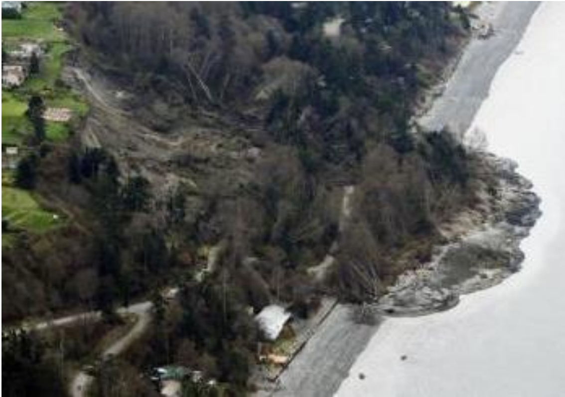
Figure 3. Oblique aerial view of the Ledgewood slide looking southward. (Seattle Times, 2013).
