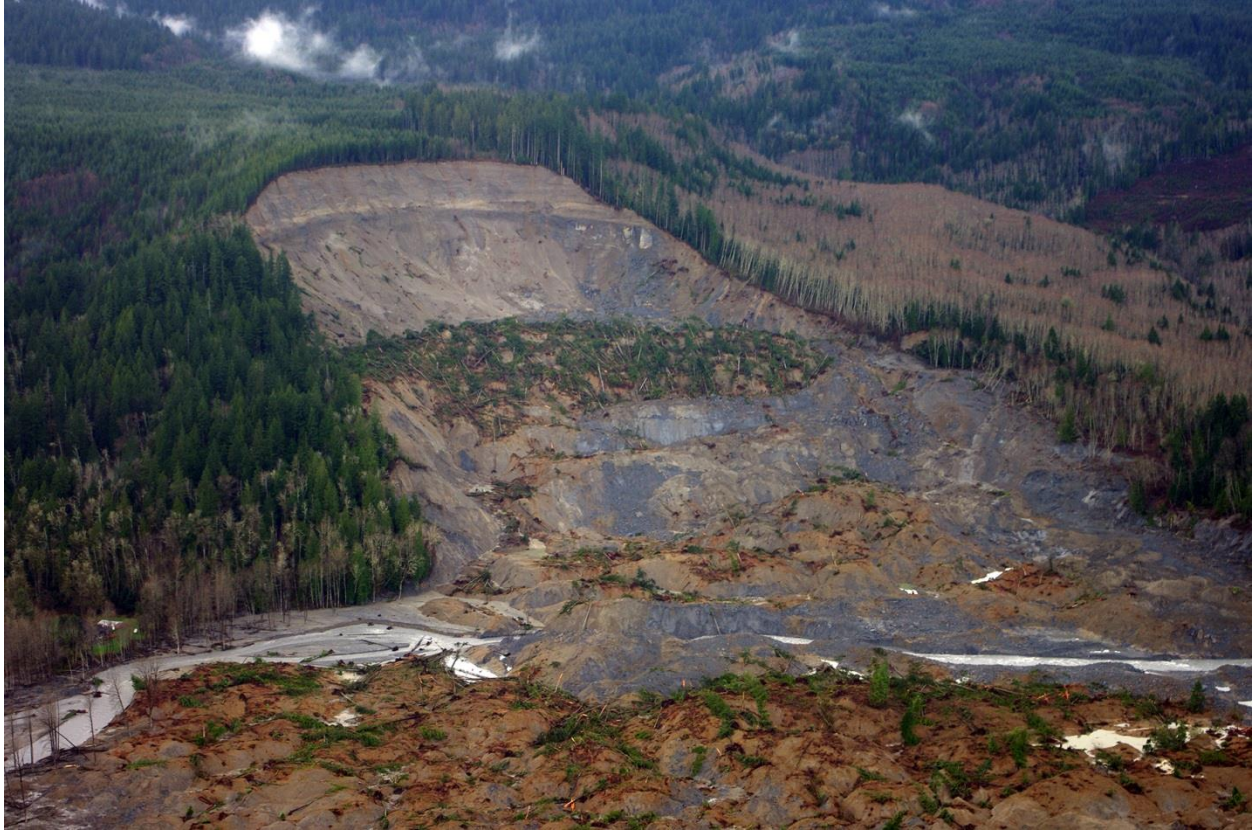
Figure 2. Oblique view of the Oso landslide looking east (Robertson, 2014). Runout from the slide can be seen crossing the North Fork of the Stillaguamish River and continuing westward out of view of the photograph. WSDOT provided the clay sample from the glaciolacustrine deposit near the base of the slope. The exact location of the sampling point is unknown to the author.
