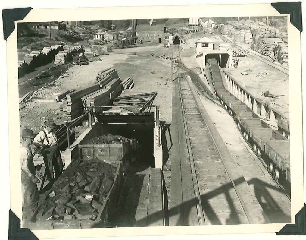
Plate XIV. Mine 3 automatic and gravity outer haulage. Loaded trips and empty trips are lifted to proper heights by the dolleys.
