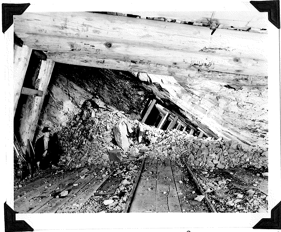
Plate V. Roslyn seam at Mine 9 on a 40^{\circ} dip. Sixteen ft timber sets on 5 ft centers. About 50 cars of rock brushed per set.
