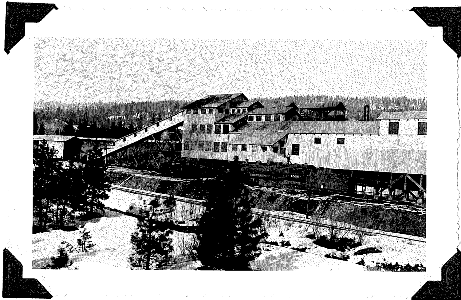
Plate XX. The central cleaning plant.
