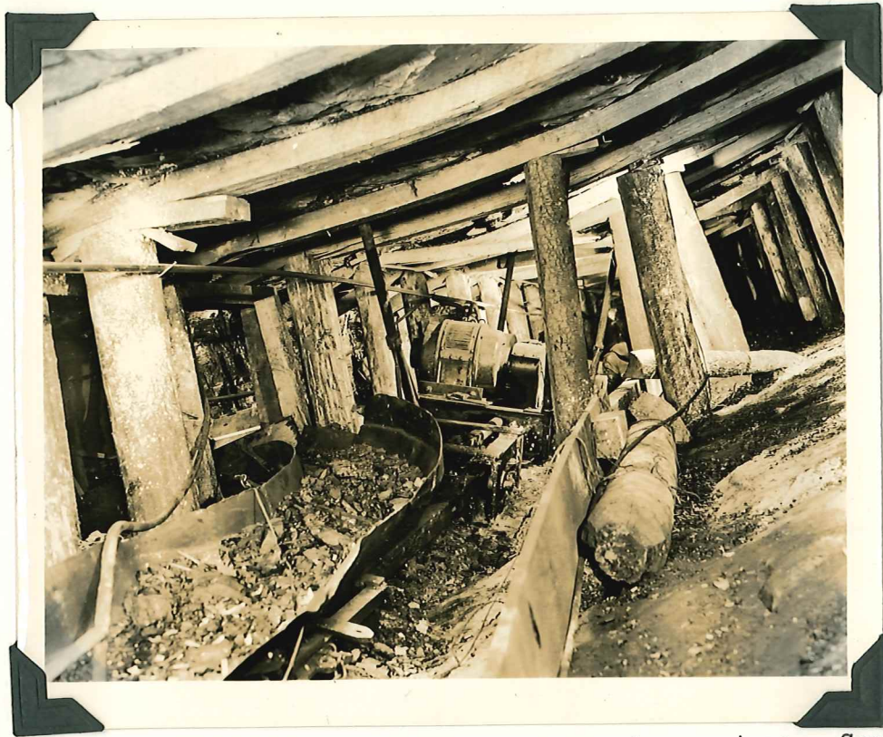
Plate IX. Underdrive conveyor in a counter entry. Conveyor discharges coal into chute which leads down through a cross-cut to the main entry. Note bottom-sniped timber.
