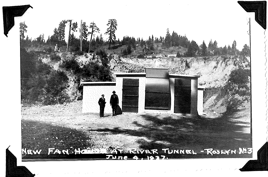
Plate XV. Mine No. 3 river tunnel fan.
