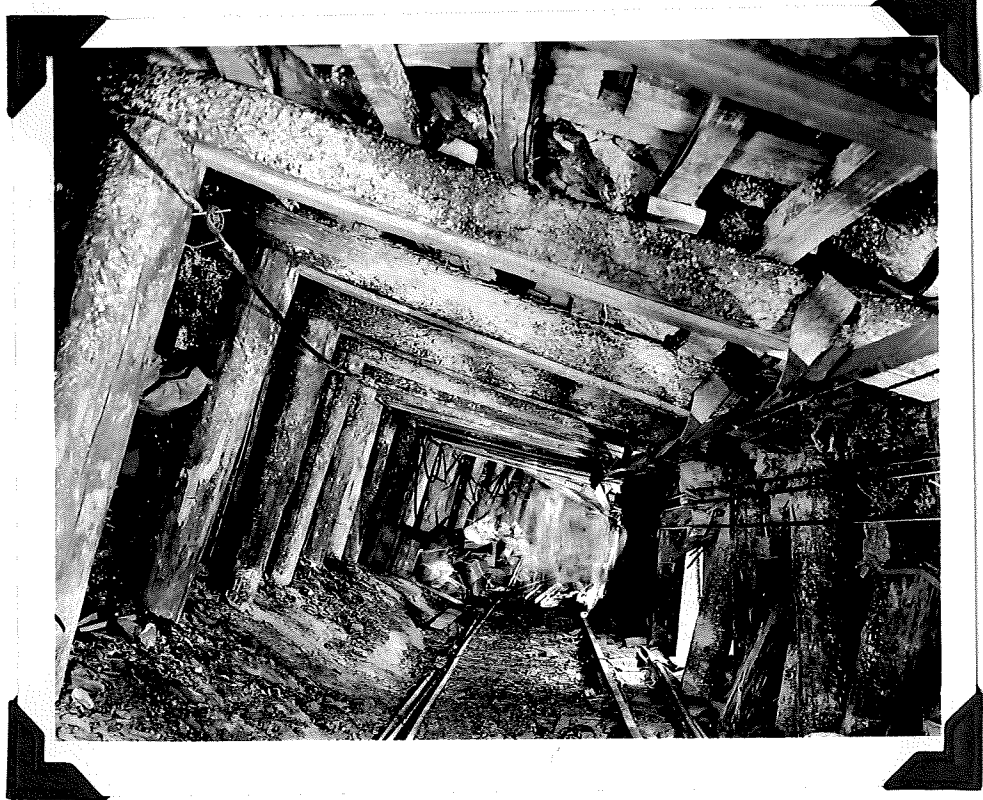
Plate IV. Mine 5 13th East permanent timbering.
