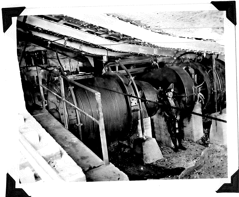
Plate XII. An underground hoist in Mine No. 3. Water rheostats, dynamic braking, and hydraulic clutches characterize this home-built hoist.
