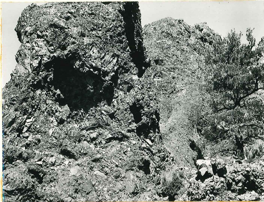
Fig. 28. View of highly fractured and in part brecciated Prospect Mountain quartzite exposed just above thrust plane which emerges along west flank of the San Francisco Mountains. Pine tree in right margin of fig. is about 20 feet high.
