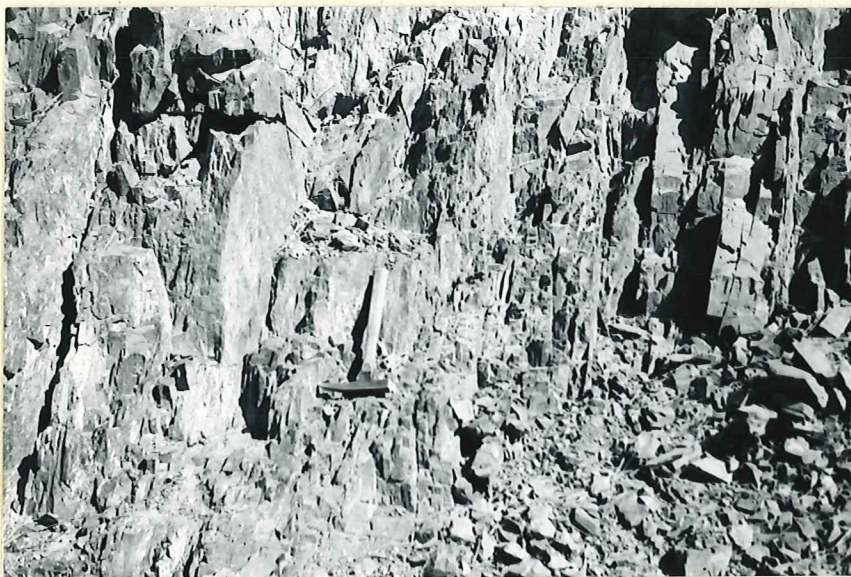
Fig. 2. Well jointed Peshastin slate from its type area on Nigger Creek.
